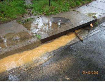
Figure 6A/B: A source of possible pollution, construction (left) and dirty water from the source entering a storm drain (right).
